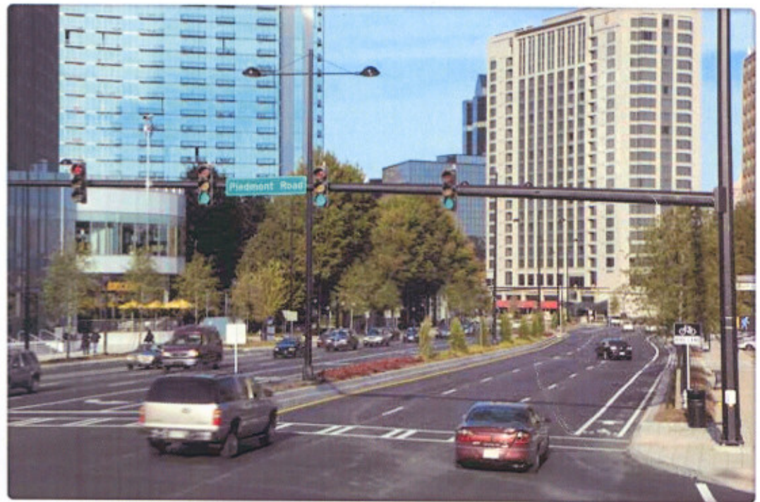
Looking north on Peachtree Road at the intersection with Piedmont Road, the features of the new boulevard are easy to see. Maintaining six lanes of moving traffic, the corridor includes wider sidewalks, new tree plantings along the curb, bicycle lanes, a center median wide enough to accommodate left turn sideslips, all utilities underground, all new street lighting and more attractive traffic signal boom arms.
